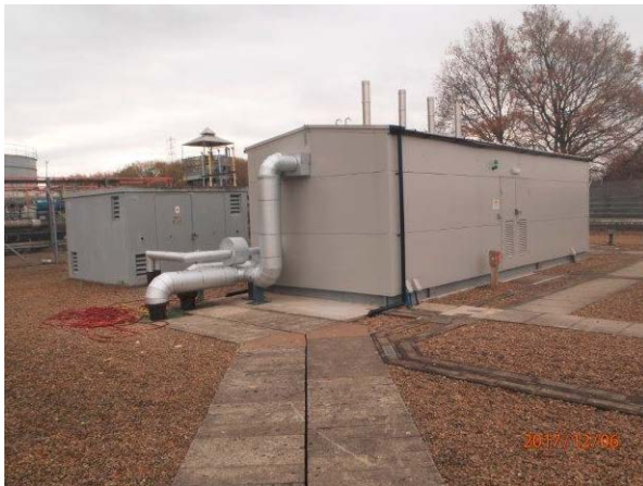
Figure 26: Existing Pathways/Ducting to the New Boiler House
