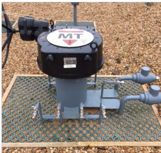
Figure 18: High Efficiency Gear Box installed at Rockland St Peter Block Valve (left); Hardwick AGI renewed (right)
