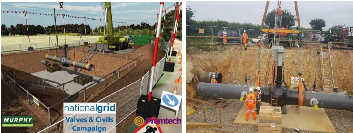
Figure 15: 3D Lifting Operation Rehearsal (left); Completed Operation (right)
