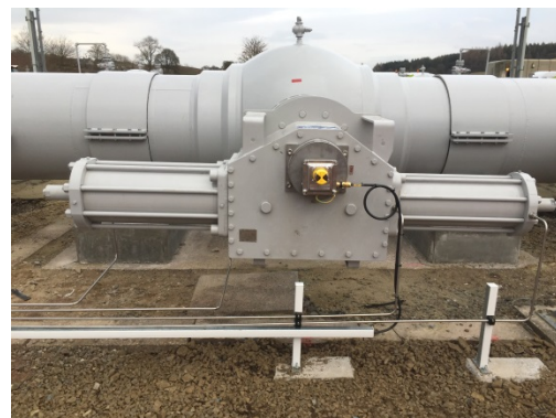
Figure 17: New Gas Actuators at Michelmersh AGI (left); New Gas Actuators at Crieff AGI (right)
