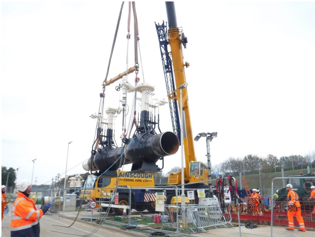
Figure 25: New pre-fabricated Perenco 1 Incomer Section commencing Installation
