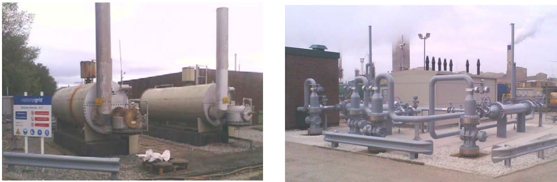
Figure 27: Left: before, Right: after
