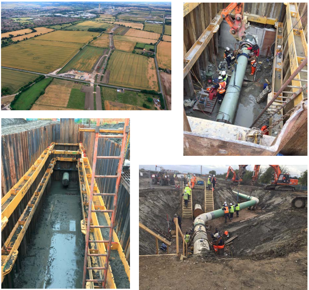
Figure 33: Diversion works at Willington Down
