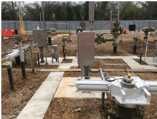
Figure 17: New Gas Actuators at Michelmersh AGI (left); New Gas Actuators at Crieff AGI (right)
